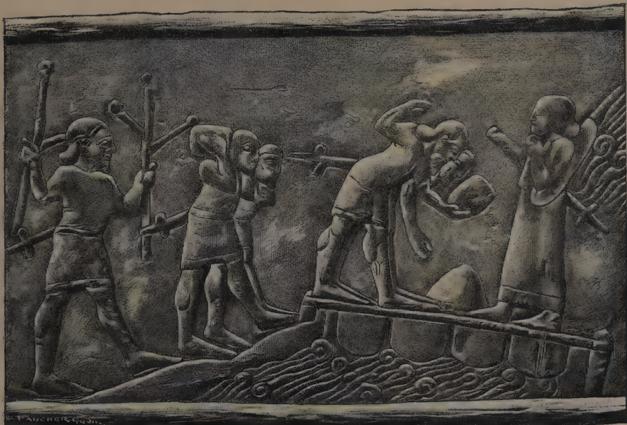
MAKING A BRIDGE FOR THE PASSAGE OF THE CHARIOTS. 1
